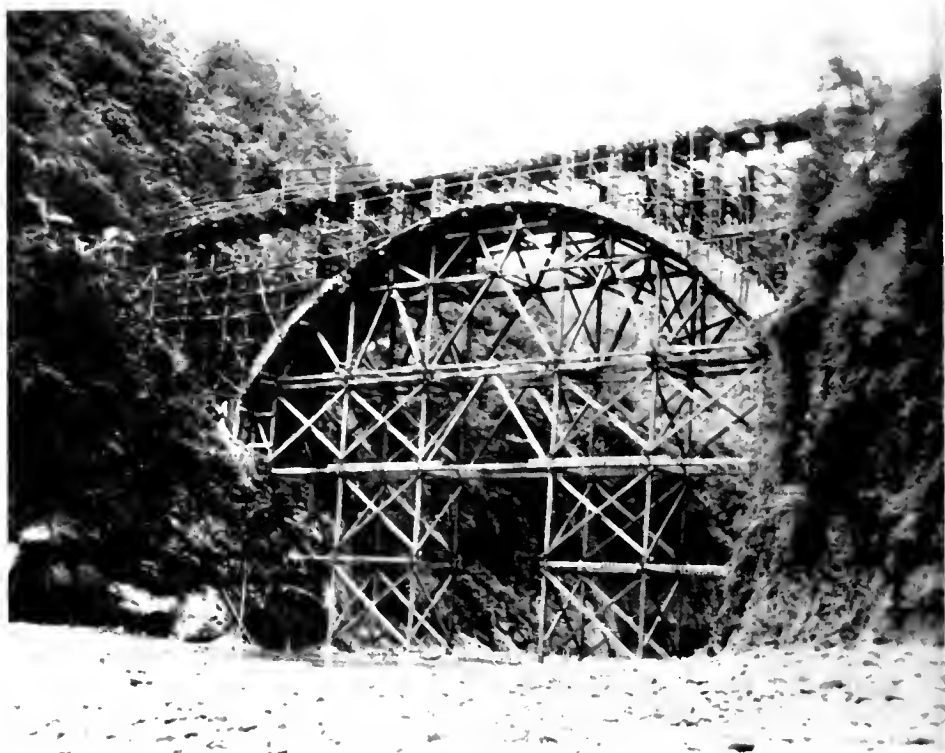
One type of arch bridge constructed in Formoso
